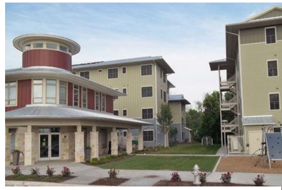
Figure 1 Austin’s M Station apartments
